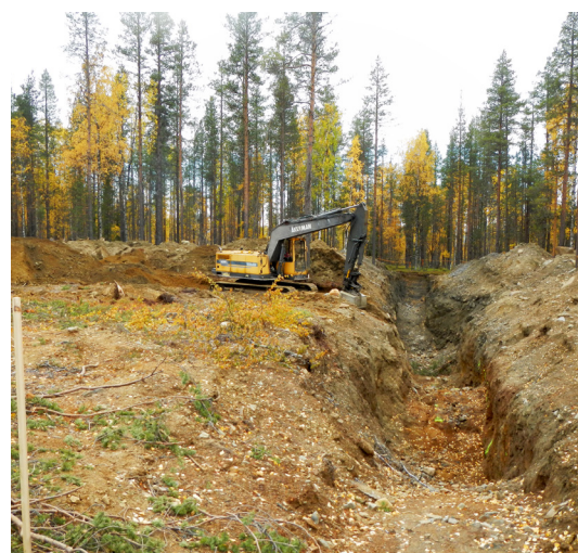
Example of exploration trench.
