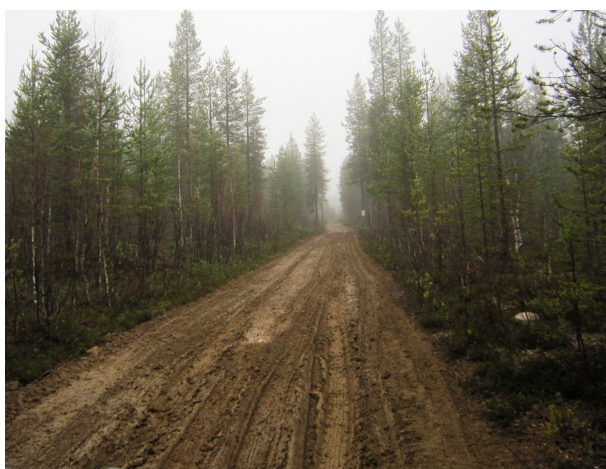
Driving damage on road without drainage. PHOTO: GEOPOOL
