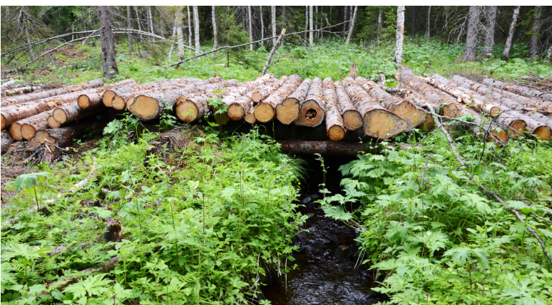
A log bridge can be constructed to allow a brook or ditch to be crossed.
