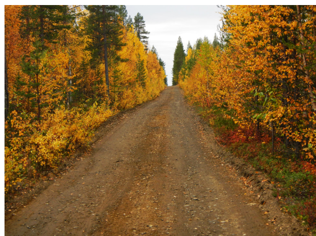
The same road after restoration, grading and backfilling.
