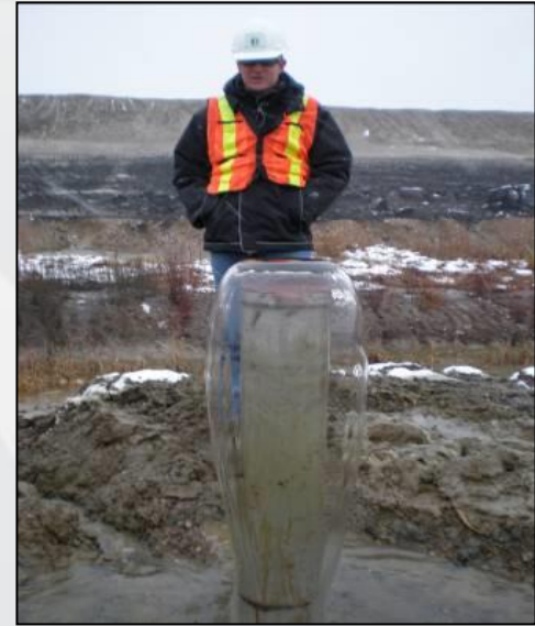
Depressurization well – artesian flow
