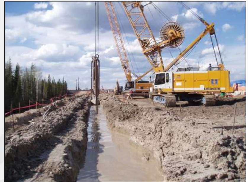
Depressurization well – artesian flow
